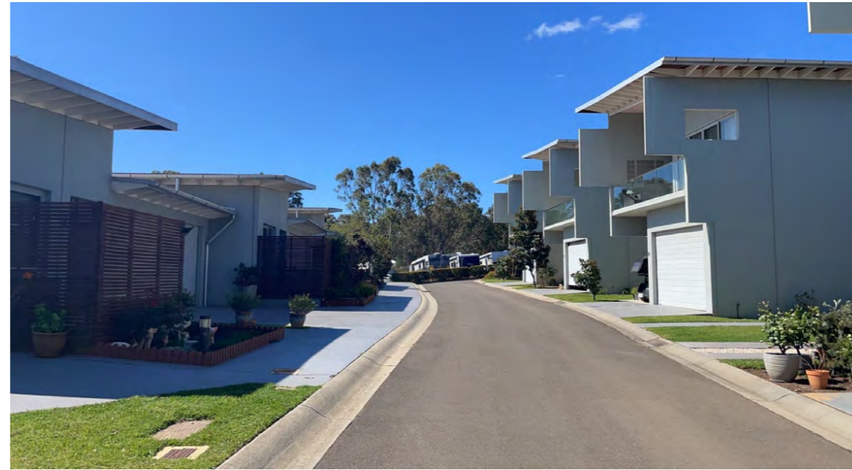
VIEW 3 - EXISTING SITE CONDITION
