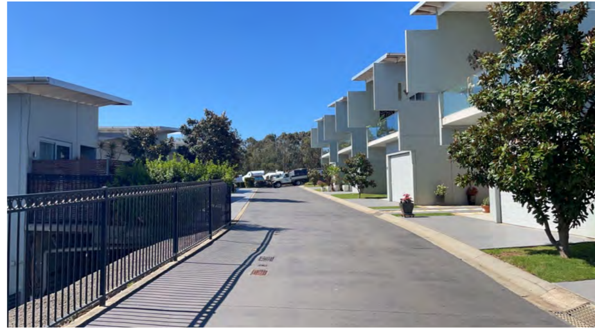
VIEW 4 - EXISTING SITE CONDITION
