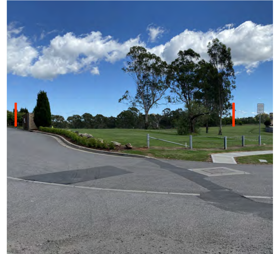
VIEW 2 - LOOKING WEST TOWARDS SITE
