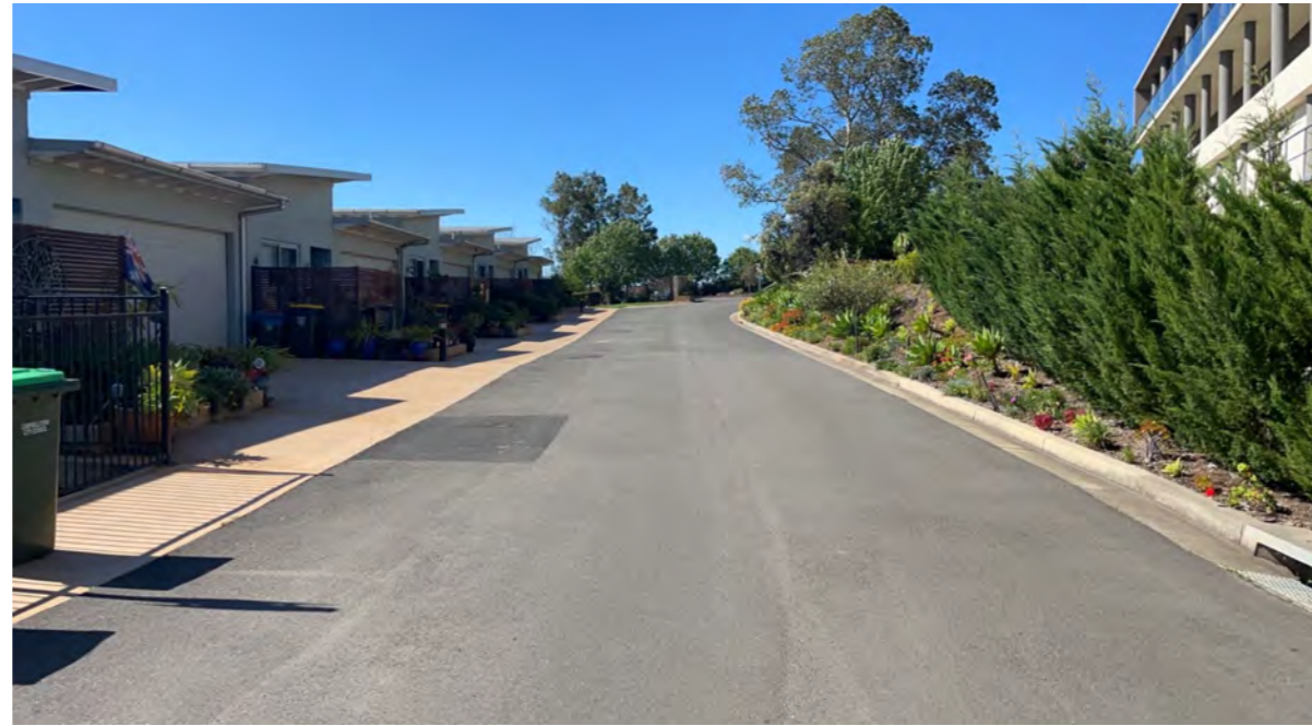
VIEW 5 - EXISTING SITE CONDITION
